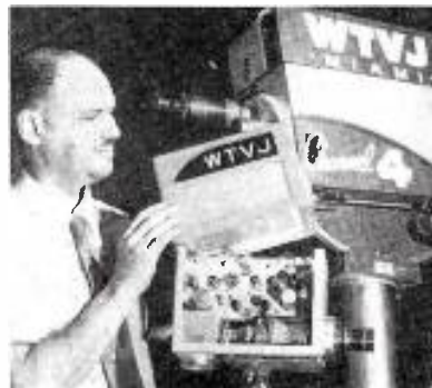
NORMAN BEAN of WTVJ (TV) Miami compares seven-pound vidicon camera which he developed for station with normal-size camera.
